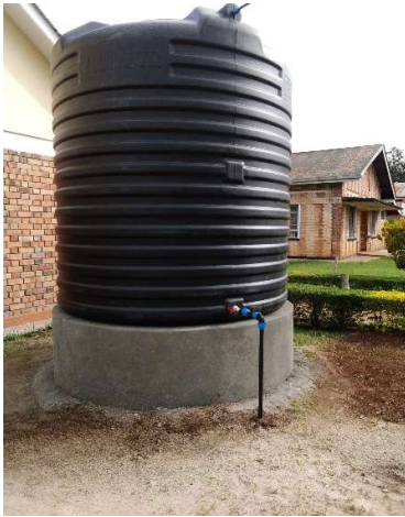
Installation 10'000 Liter Tank
